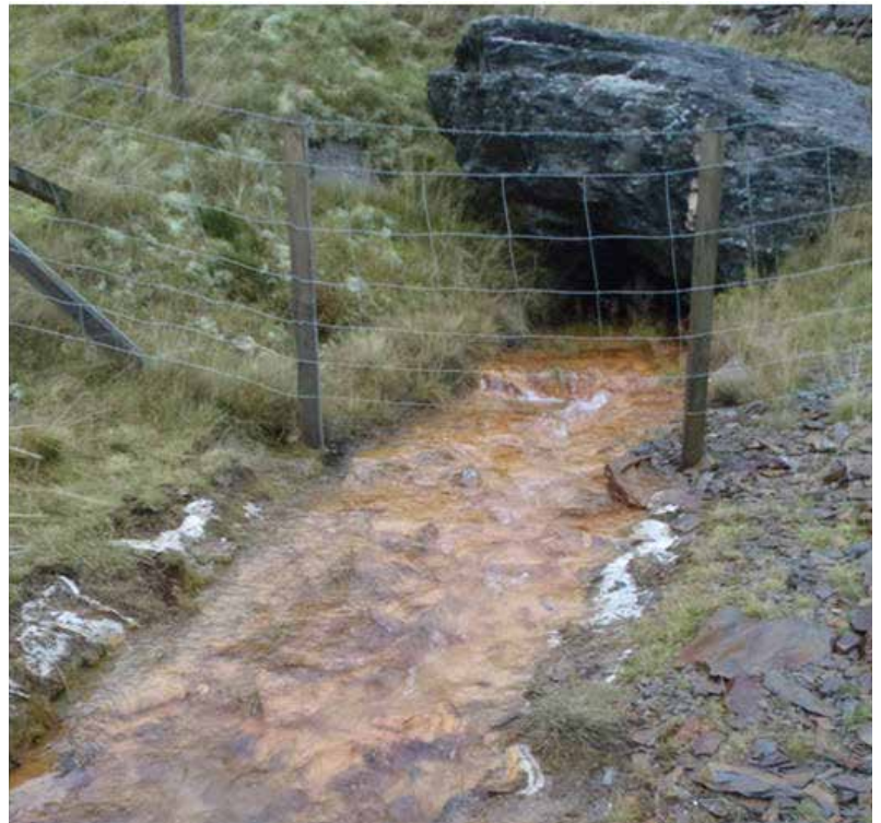
Figure 2 Field evidence of metal precipitation in the form of iron ochre at Pugh's adit, a point source, but also where zinc attenuation is occurring.
