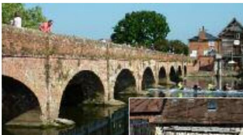
The canal linking the River Avon to Birmingham was completed (1816) thanks to transport entrepreneur William James. He owned the Wilmcote quarries, and realised how much easier it had been to lay rails in his quarries than to dig the canal. So he built this fine brick bridge (1826), and the tramway to Moreton-in-Marsh, to transport coal, machinery and agricultural products between the Black Country and the Cotwolds via Stratford. The relatively new wall behind the railway wagon is of Blue Lias.
