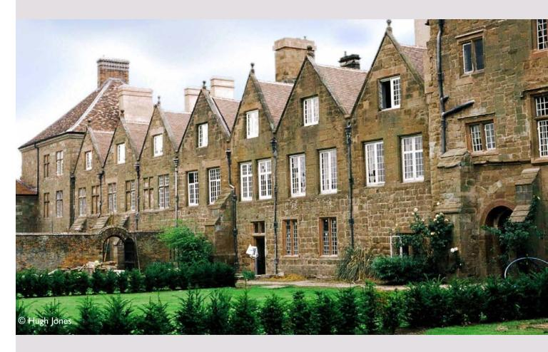
At Stoneleigh Abbey part of this substantial stone building is constructed of red Kenilworth Sandstone (east wing top image) while in contrast the principal façade of the west wing (bottom image) is constructed of pale grey Bromsgrove Sandstone. Recent restoration work on the west wing has used white Triassic Grinshill stone for major repairs. At Stoneleigh village, locally quarried sandstone from Motslow Hill is displayed in the almshouses.
