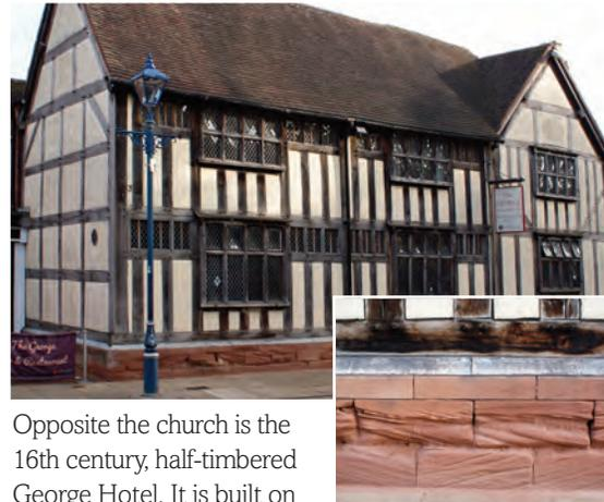
Opposite the church is the 16th century, half-timbered George Hotel. It is built on a foundation of sandstone, that exhibits the layering of sediments showing they were laid down in rivers
