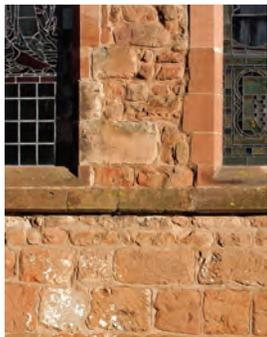
The rubble stone walls of the early chancel contrast with the dressed stonework of the later nave. Rubble stone is easily obtained from the top metre or so of a quarry whereas deeper levels provide better quality 'freestone', suitable for squaring and dressing, and called ashlar.
