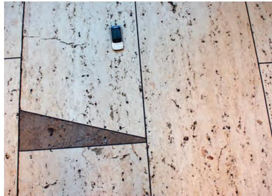
travertine. **Travertine** is a form of limestone precipitated from hot mineral springs. Darker colours in the stone result from impurities such as iron and copper. The stone takes its name from Tivoli near Rome and was used extensively by the Romans for temples and other public buildings.
