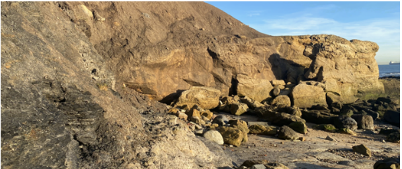
The NFD fault plane, its only surface exposure is here at Tynemouth North Point. The Westphalian coal seam with seat earth (fireclay) below can be easily seen to the left side. With the wavecut platform to lower right. Glacial till caps this outcrop.
