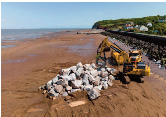
Rock armour on the beach at Blue Anchor during a previous temporary job that was carried out in 2022. (Image Aggregate UK)
