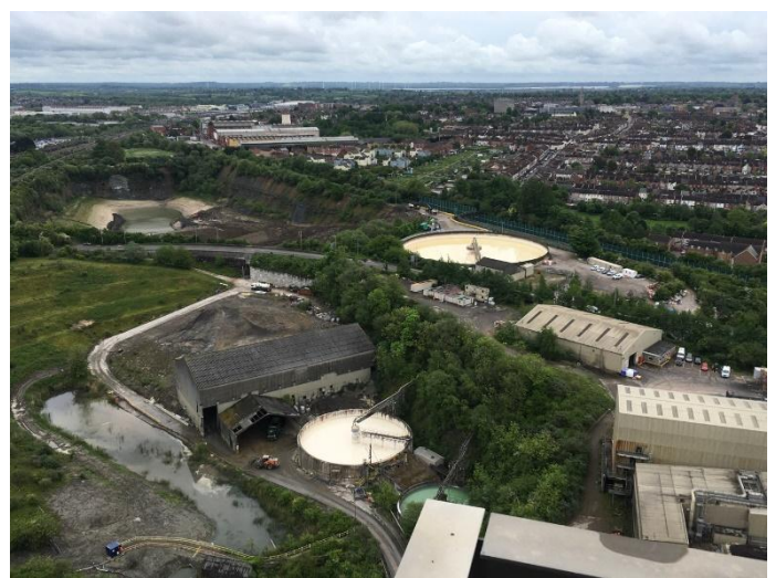
View from gantry over CEMEX Rugby and old clay quarry
