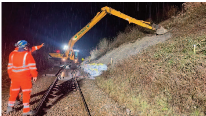
Over a thousand tonnes of material had to be moved. (Image: Network Rail)
