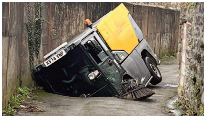
A giant sinkhole at Rhondda Cynon Taf, which buried this road, and sweeper. (Image: Local handout)
