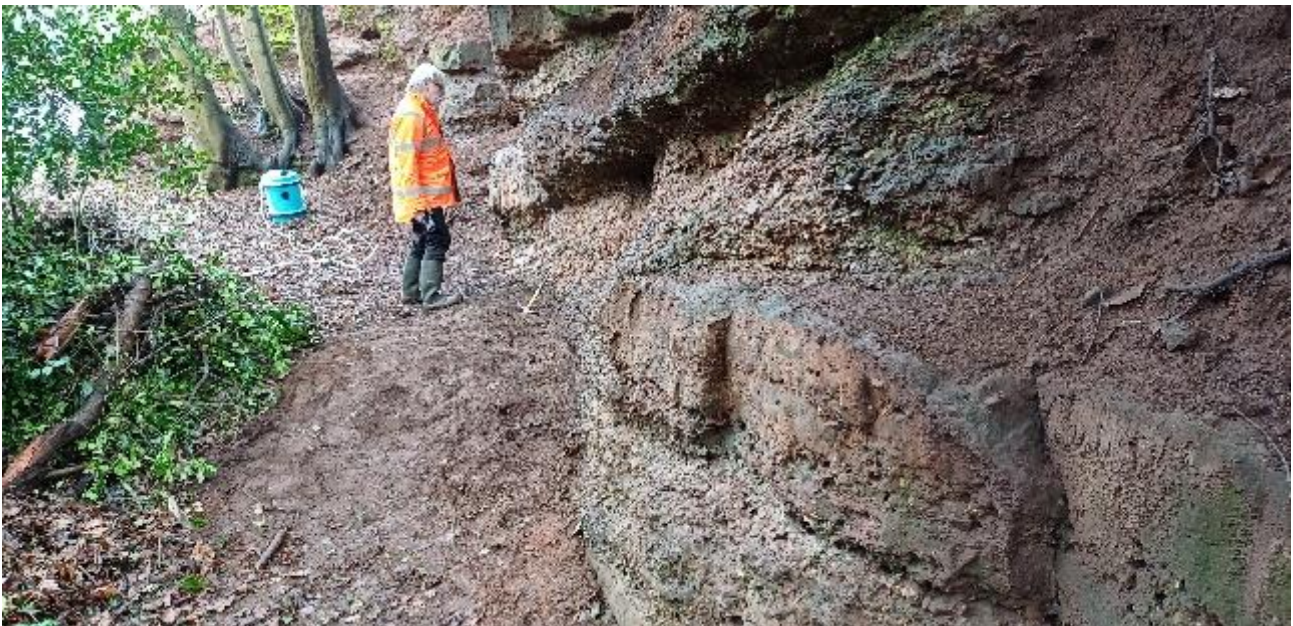
A small group of WGCG members have diligently spent time cleaning the quarry faces to reveal its geological features and clearing the access routes to this geological gem within our LGS portfolio
