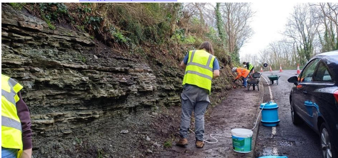
Volunteers clearing the vegetation and soil from the exposure and footpath prior to jet washing.
