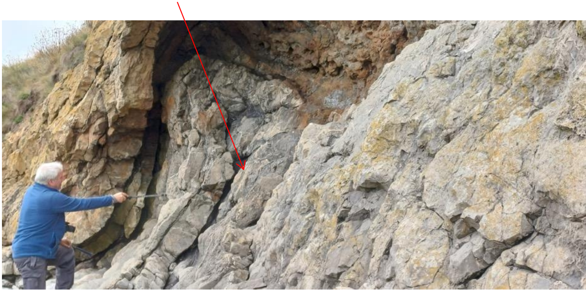
Overfold. The red arrow points to an "upside down" limb
