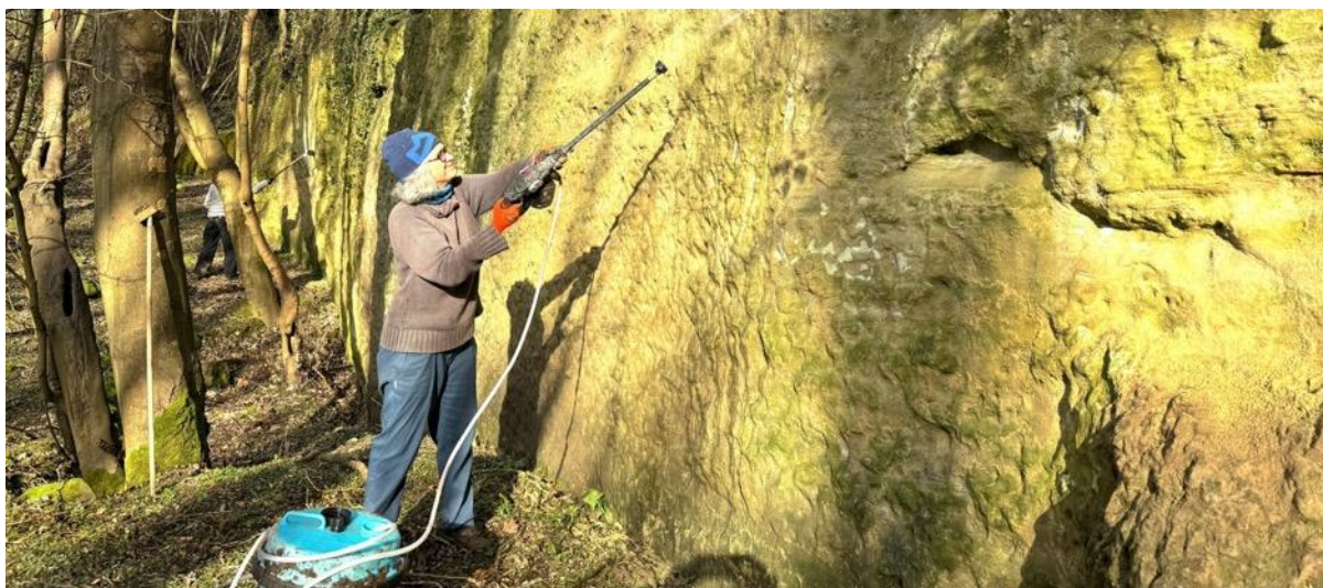
Cleaning the quarry faces with the mobile jet wash and wire brushing
