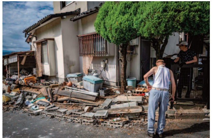
A house collapsed after an earthquake in Yatsushiro, Kumamoto Prefecture, Japan, on the 28th.
