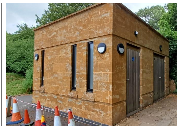
Figure 39: New toilet block by All Saints Church
