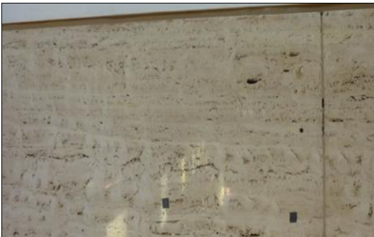
Figure 16: The Core Exterior
